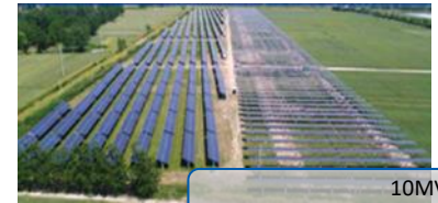
10MW Jiangsu, China
