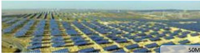
50MW Datong, China
